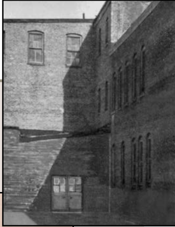
Longworth St. Original Location (1907 - 1910)
